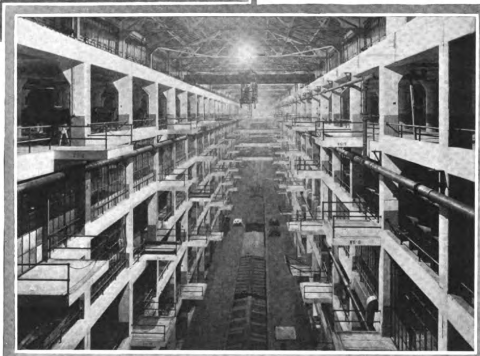
Below—A view in the six-story shipping building, showing some of the 204 loading platforms
